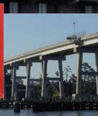
Sneads Ferry Bridge
